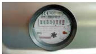
The **water meter** measures the water flow at the inlet. This is particularly important for the combination pre-filter, as it must be replaced after approx. 30,000l.
